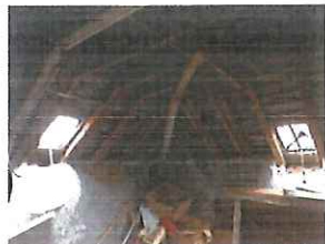
Grenier 24,8m 2 (charpente sans isolation)
